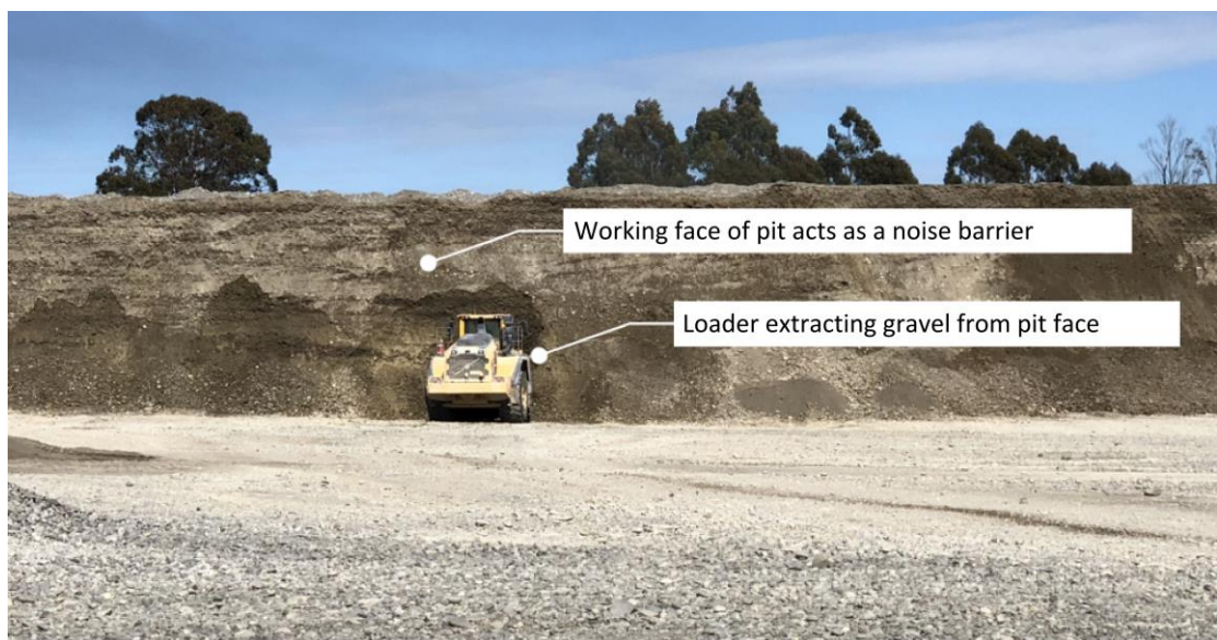
Figure 2: Example of loader activity at edge of pit
