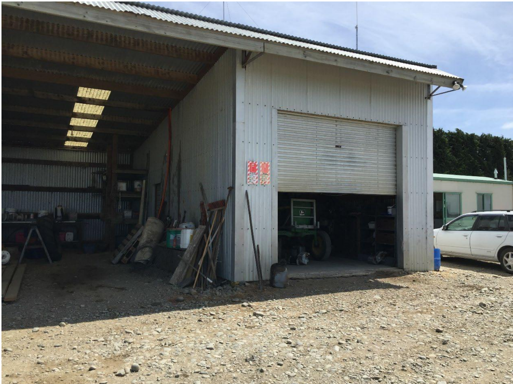
Photograph 4: (View of the northern side of the barn and mechanics workshop)
