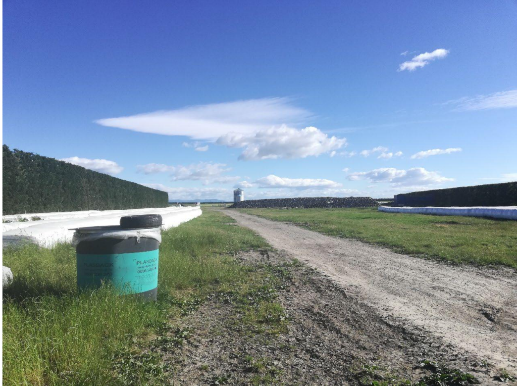
Photograph 1: (View north from the yard looking towards the silos)
