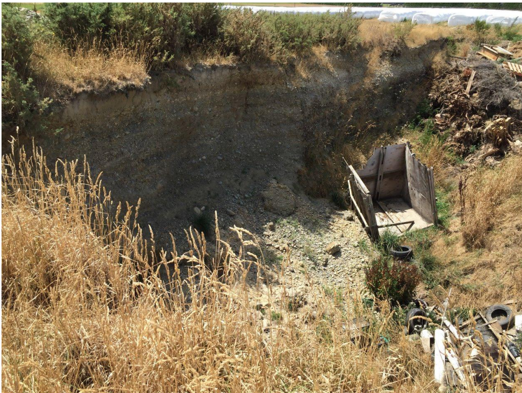
Photograph 6: (Current waste pit looking north-east, showing soil profile on northern edge of pit and waste material including wood, organics and tyres)
