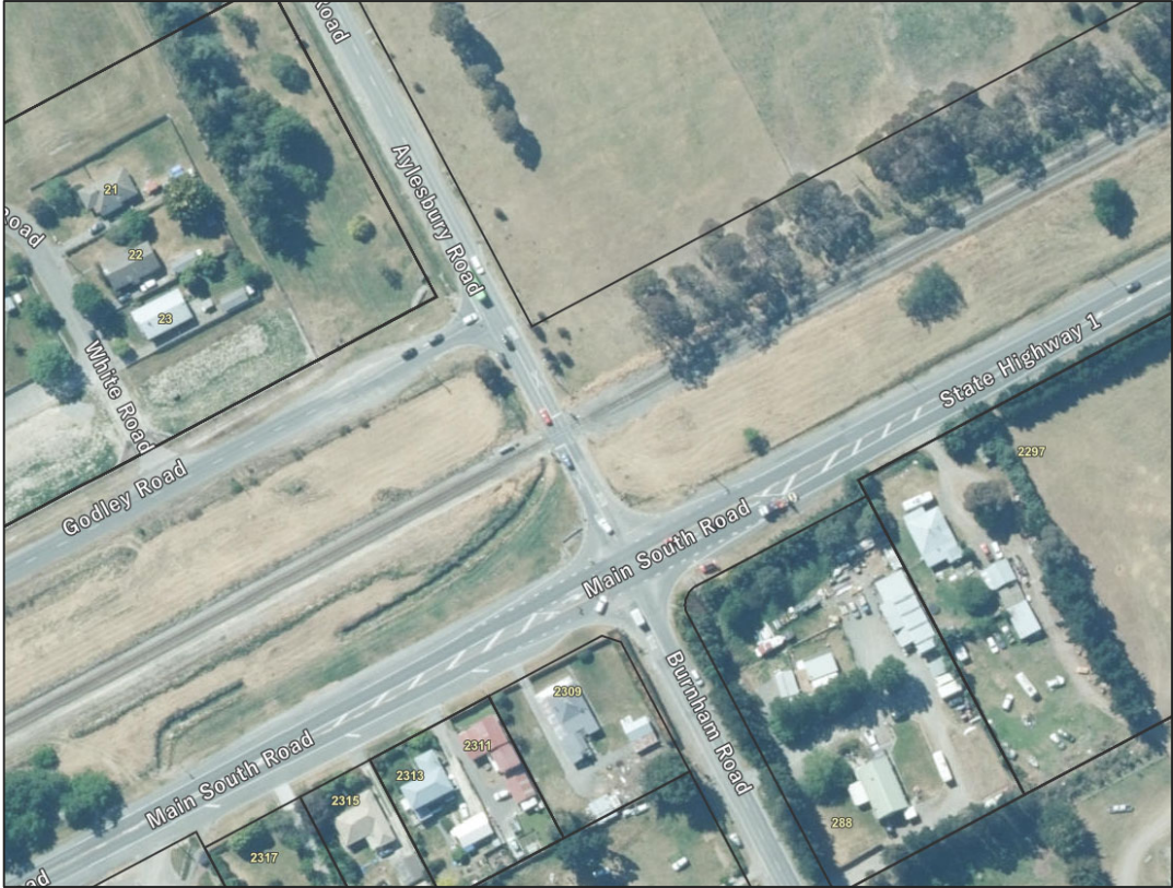
Figure 3-7: Aerial Photo of Aylesbury Road and SH1 Intersection (Canterbury Maps)
