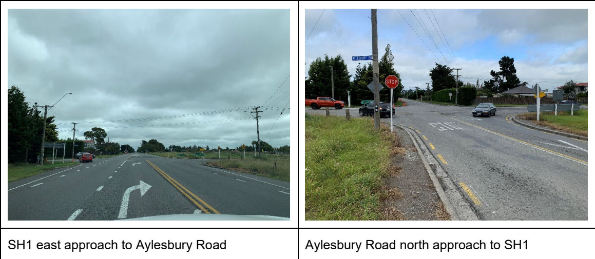
Figure 3-8: Photos of SH1 / Aylesbury Road
