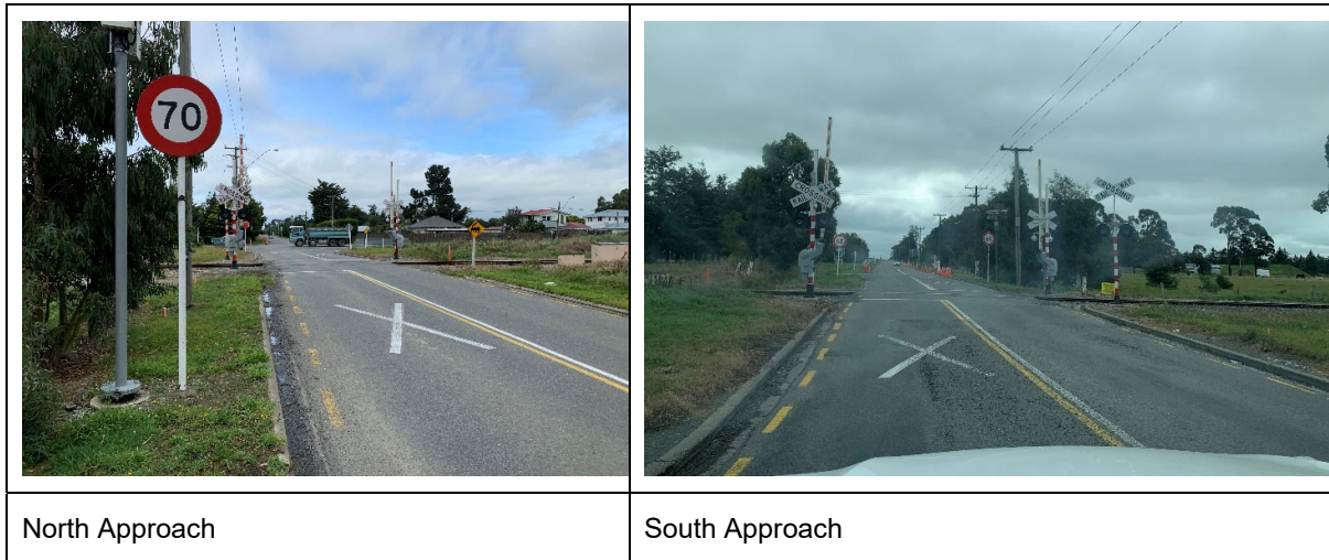
Figure 3-9: Photos of Aylesbury Road Railway Level Crossing
